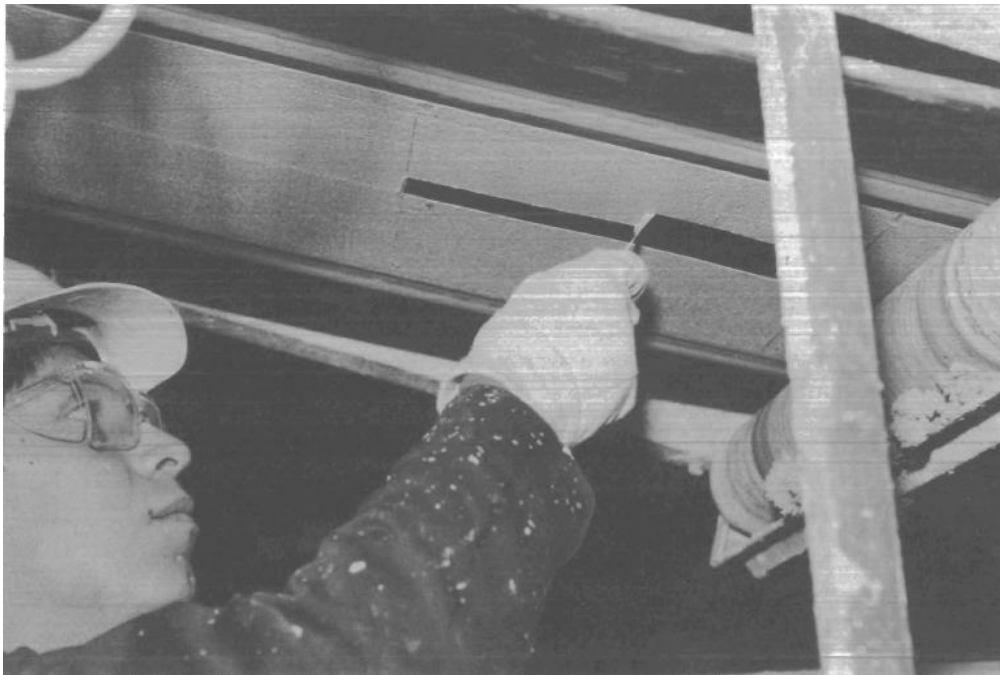
Figure 54: Fine material stuck to conveyor belt (from [19] in public domain)
